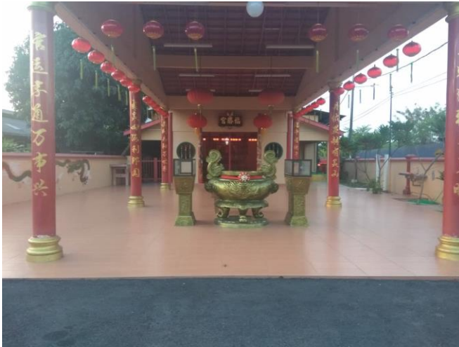
Figure 4: One of the Taoist Temple in Tanjung Kling, Fu Sheng Gong
